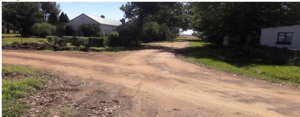
Image 3: Untarred Roads in Urban Residential Area
